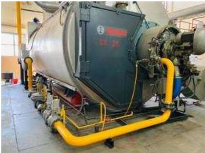
Conversion of boiler fuel for its Green Leaf Threshing Plant's operation from furnace oil to Liquefied Petroleum Gas (LPG) which is expected to reduce CO2 emissions by **30%** which translates into a reduction of 2200 tons of carbon emissions in the next five years
