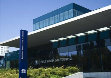
HQ (Operation Center) at Switzerland/Lausanne
