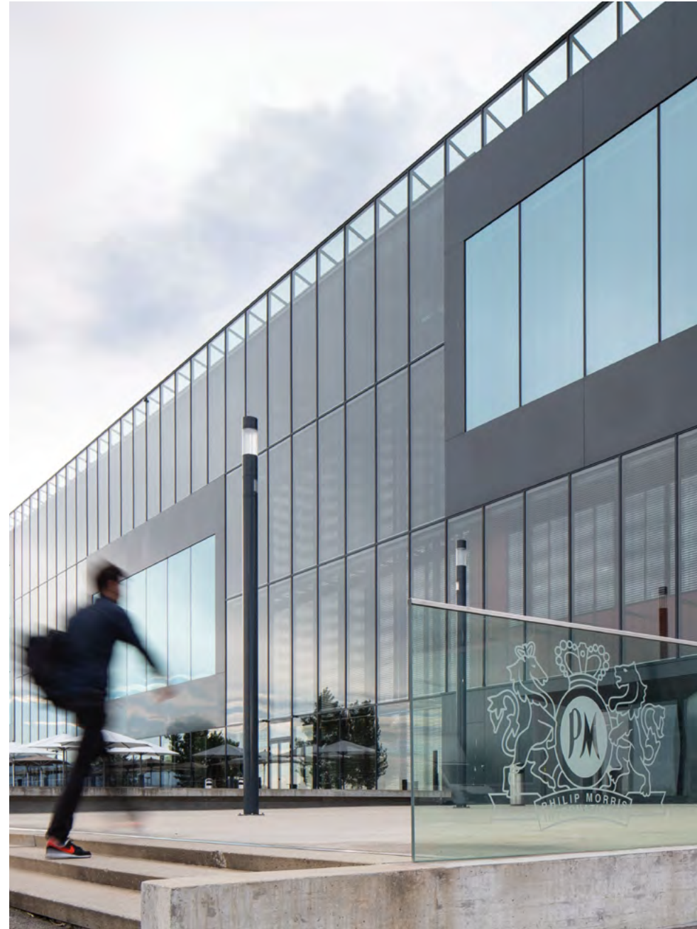
PMI's R&D center in Neuchâtel, Switzerland
