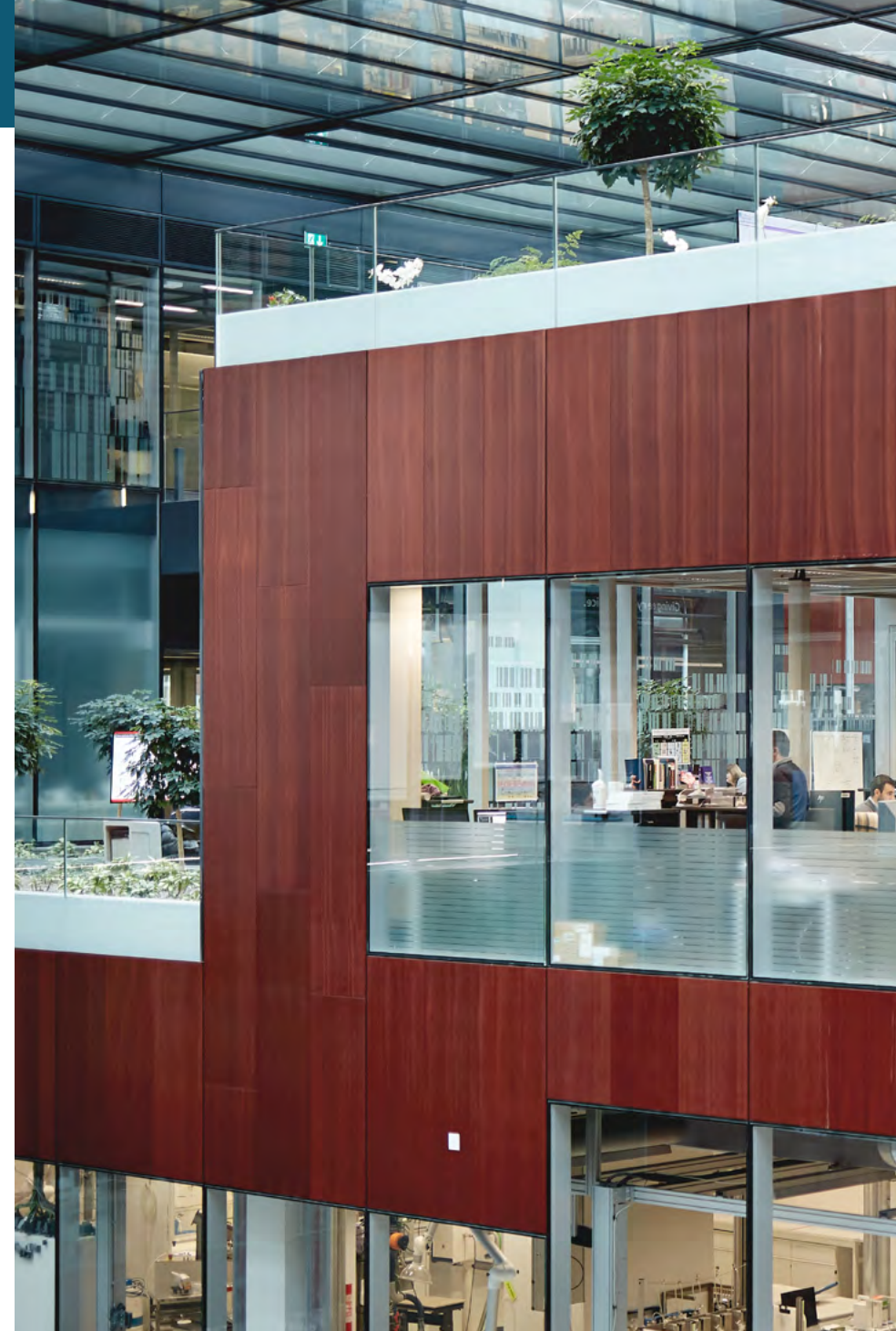
PMI’s R&D center in Neuchâtel, Switzerland
