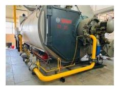
Conversion of boiler fuel for its Green Leaf Threshing Plant's operation from furnace oil to Liquified Petroleum Gas (LPG) which is expected to reduce CO2 emissions by 30% which translates into a reduction of 2200 tons of carbon emissions in the next five years
