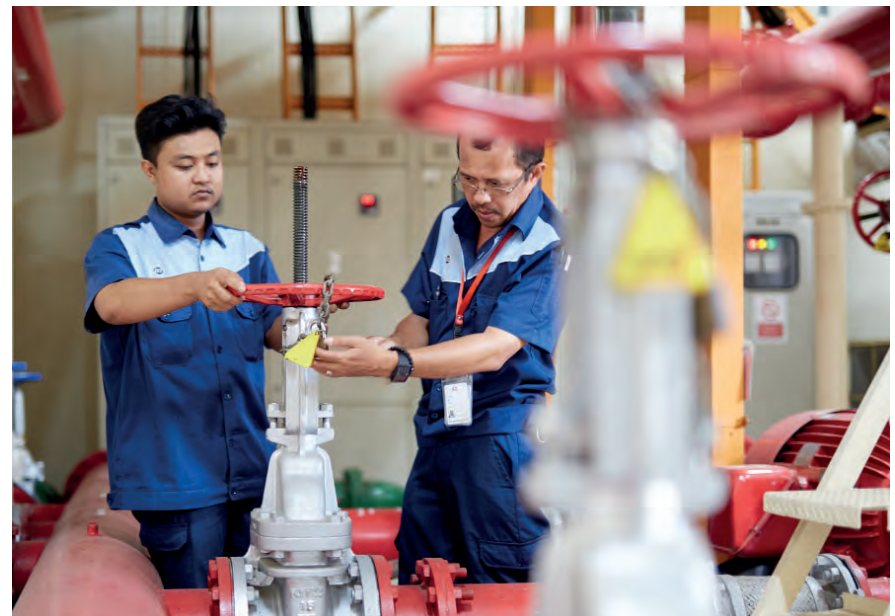
Above: Wastewater treatment in PMI's Indonesian affiliate Sampoerna's manufacturing facility in Sukorejo
