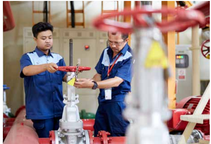
Above: Wastewater treatment in PMI's Indonesian affiliate Sampoerna's manufacturing facility in Sukorejo
